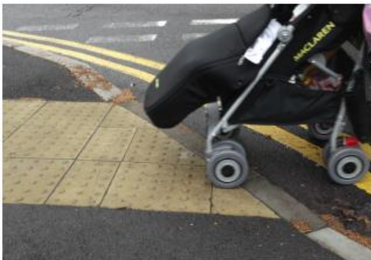
Dropped kerb with tactile paving
