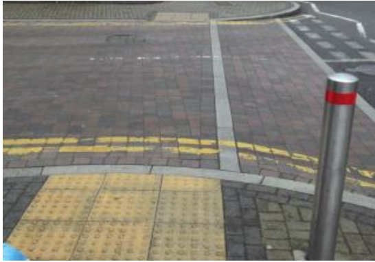
Side road entry treatment and speed table
